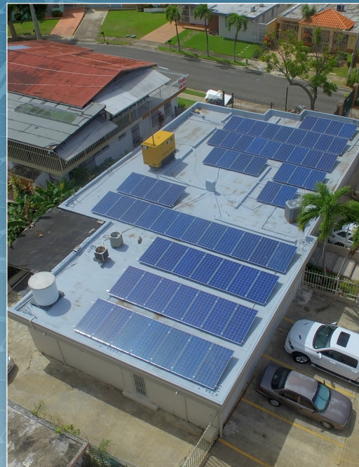
15 kw Commercial System, Guaynabo
